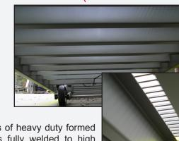
Structure consists of heavy duty formed steel side girders fully welded to high strength steel joists. (Picture shows under side of ramp)
